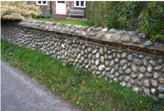
Flint cobble wall
