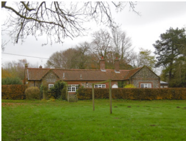
The Old School Room
