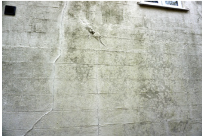
Cracked render and dirty paintwork
