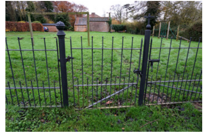
Metal gate and railings to the graveyard
