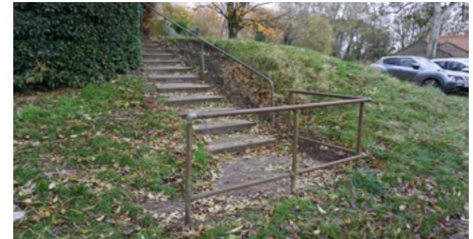
Utilitarian tubular railings
