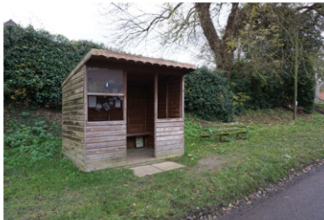
Bus shelter in poor decorative condition
