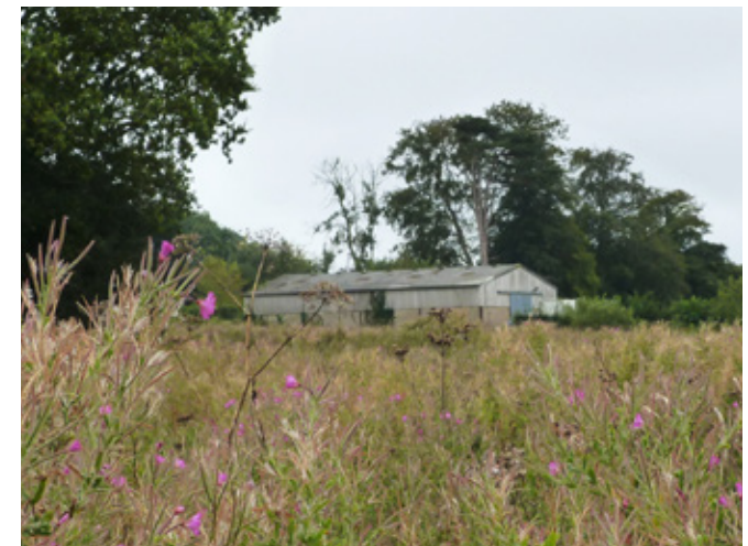
Modern agricultural barn seen on the edges of the Conservation Area from the surrounding fields
